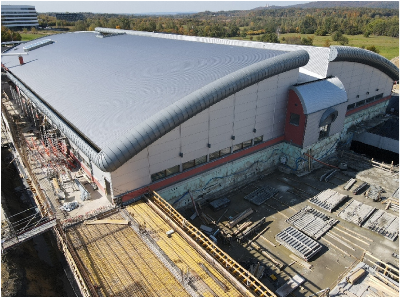
Construction work at SOLARIS (photo: Krzysztof Adamczyk)
